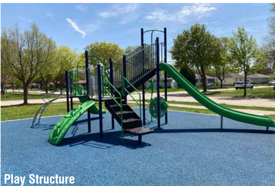
Poured-in-Place Play Surfacing
